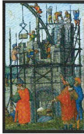
fig. 9 "Scaffolding & Centering", How to Build a Cathedral , Hislop, Malcolm, p135
