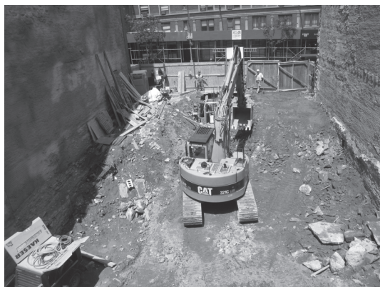
At 39th & Lexington in Midtown Manhattan, our client's neighbor, building a 33 story hi-rise, we supervised the underpinning of client's 5 story office building in 2015 with the guidance of same engineering firm for the World Trade Center, MRCE.
